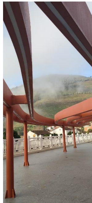
Figure 2. “Pinhão” Village—The Douro Wine Region (Credits by the author).
