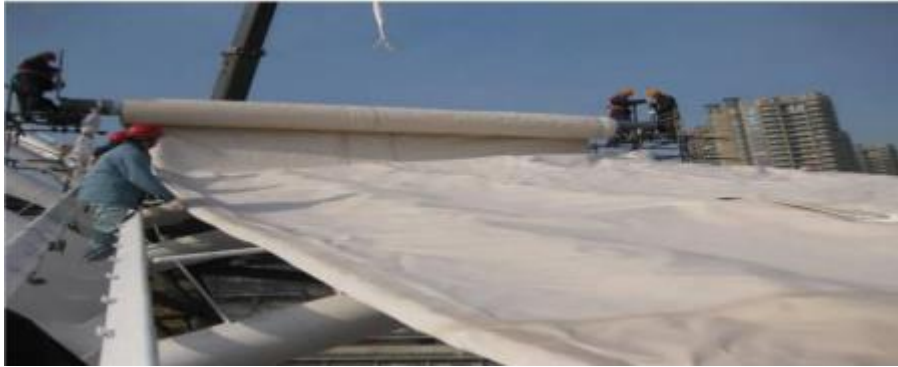
Figure 4 Schematic diagram of membrane spreading.
