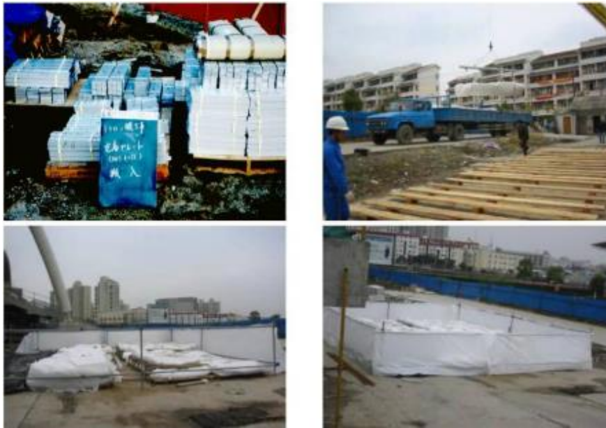
Figure 3 On-site membrane material yard.
