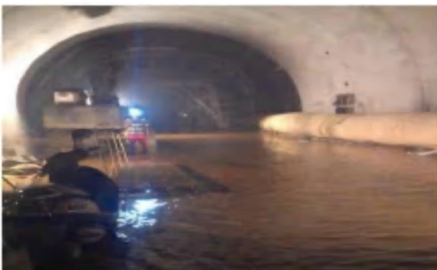
Figure 3 Surface collapse in muddy and watery areas.
