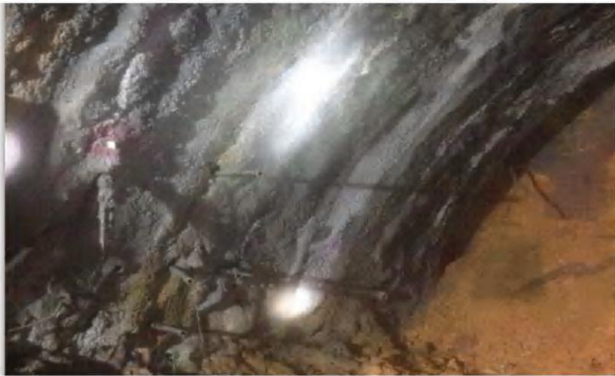
Figure 11 Radial supplementary grouting construction.
