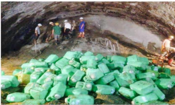
Figure 13 Weideke chemical slurry supplementary grouting.
