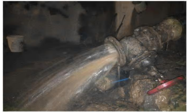
Figure 14 Drilling drainage holes for water diversion and drainage.
