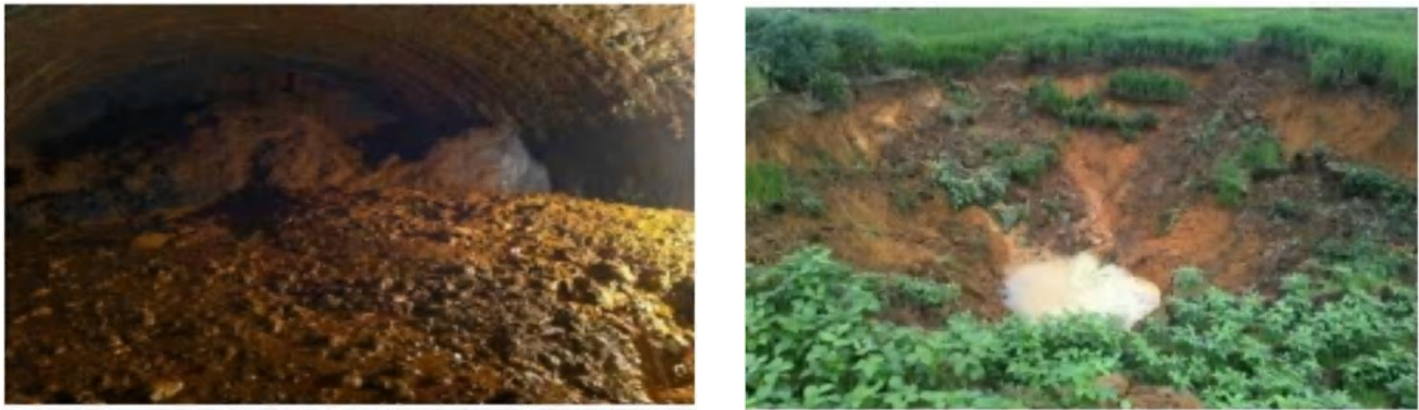
Figure 4 Surface collapse of Tu Ni Yao.
