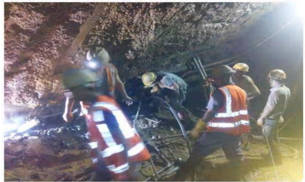
Figure 12 Construction of large lock foot drilling and grouting.
