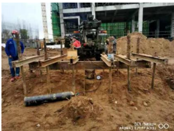
Figure 14 Pictures of on-site testing (III).
