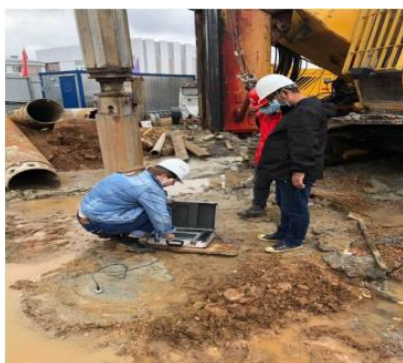
Figure 12 Pictures of on-site testing (I).
