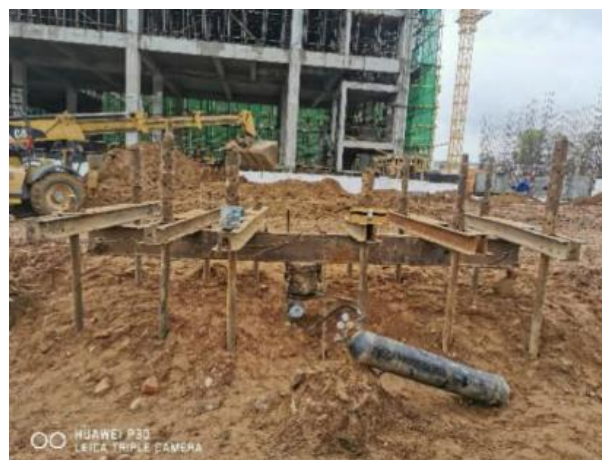
Figure 15 Pictures of on-site testing (IV).
