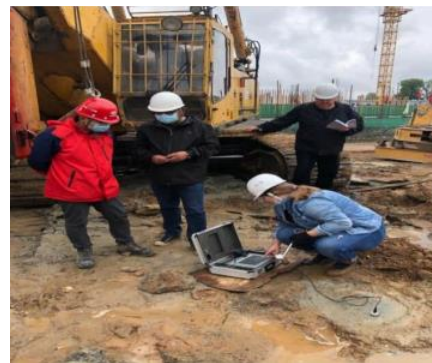
Figure 13 Pictures of on-site testing (II).
