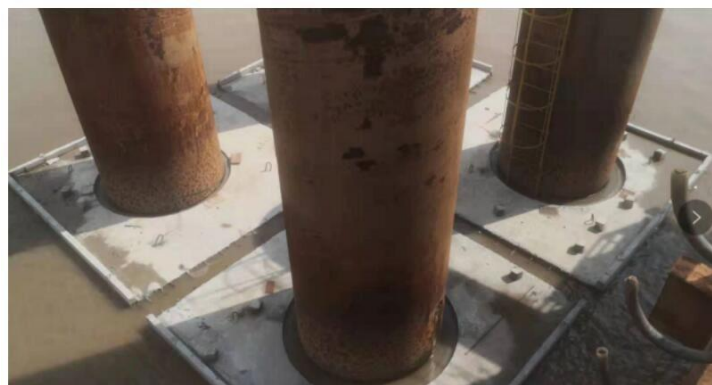
Figure 9 Prefabricated bottom plate assembly site diagram.
