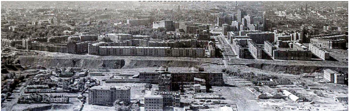
Figure 3. The Shatilovsky Yar ravine in the middle of the photo (early 1930s). The ravine was 10 m deep. It was subsequently filled with construction waste and displaced soil.
