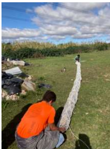
Figure 1. Biofence built and installed in the Chacarita stream.
