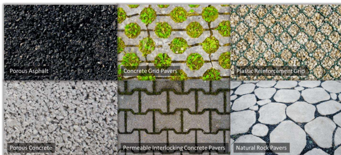
Figure 5. Types of permeable pavements [62] .
