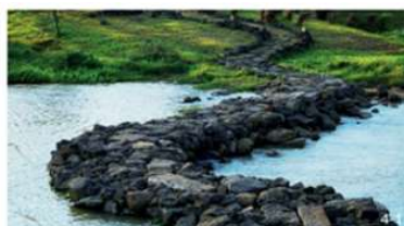
Figure 4-1. Volcanic stone snake bridge after completion.
