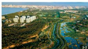
Figure 3-2. Real picture after restoration.
