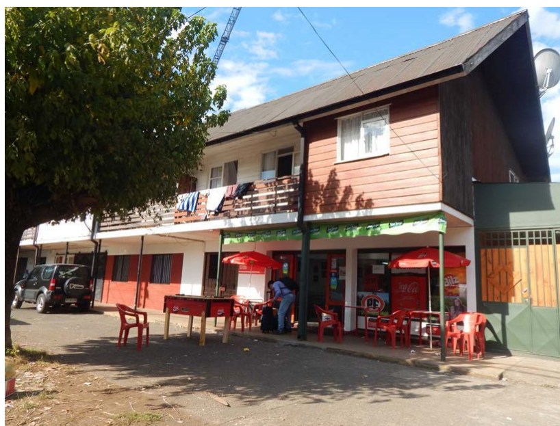
Figure 5. The house continues to be commercially renovated on the first floor.
