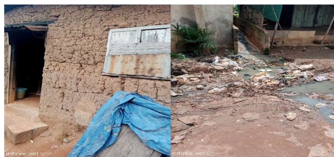
Figure 4. Building and road condition in Ugbo-owa.
