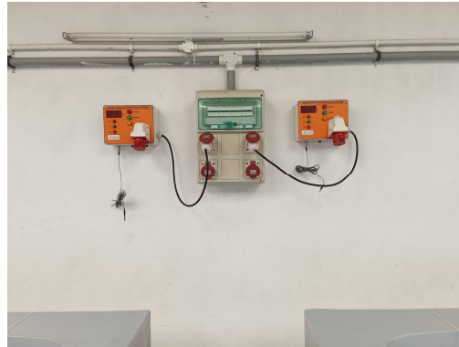
Figure 3. A closer view of the installed device.
